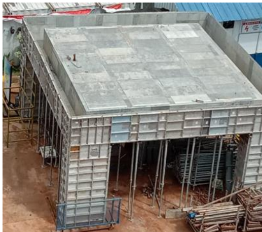
Fig. 1 Aluminum Formwork
