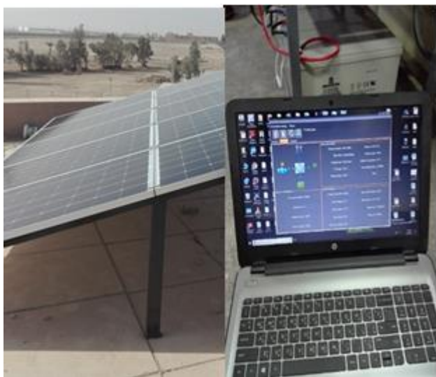
Figure 5. Piratical installation of solar photovoltaic systems (PV) Off Grid.
