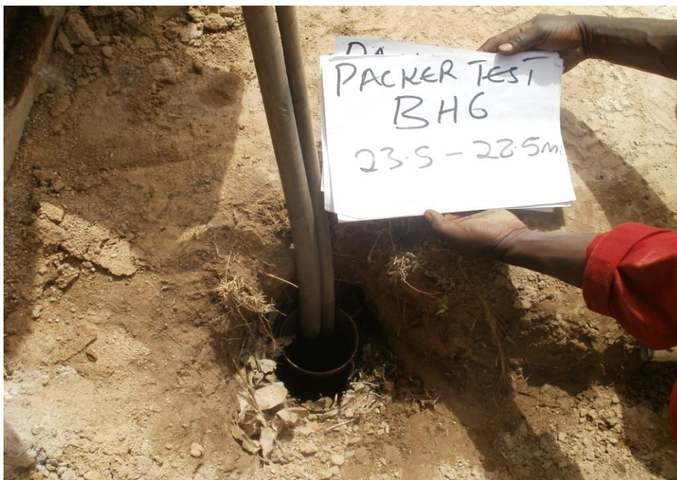
Figure 8. Pumping in progress through the packer tube
