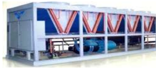
Fig1: V configuration condenser coils
