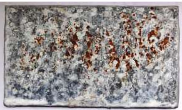
Figure 7 : Photograph of salt spray test Galvanised steel after 1200 hours.
